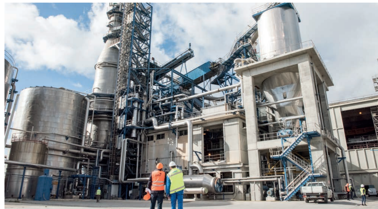
ANDRITZ supplied the latest technology for the digester and chip feeding system at Celbi.
